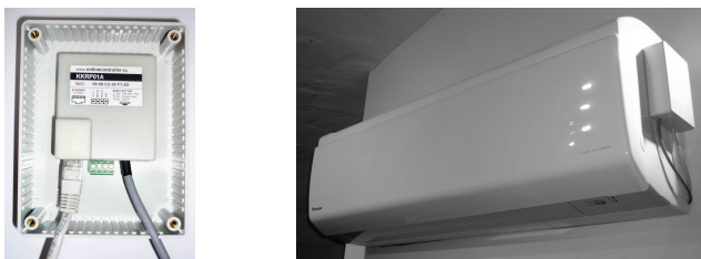
Figure 3 – Installation examples of the KKR01A adaptor
